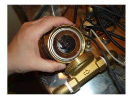
Now, the rotor ball in the interior of the pump becomes visible.
