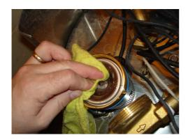
The pump housing should also be cleaned. Then place the clean rotor ball back into the housing.
